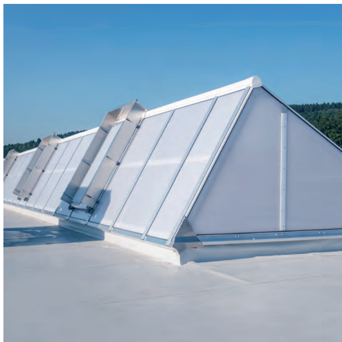
LAMILUX Continuous Rooflight S on the industrial hall of Kemper GmbH in Olpe
