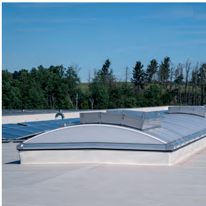
LAMILUX Continuous Rooflight B on the industrial hall of Bang Kransysteme in Oelsnitz
