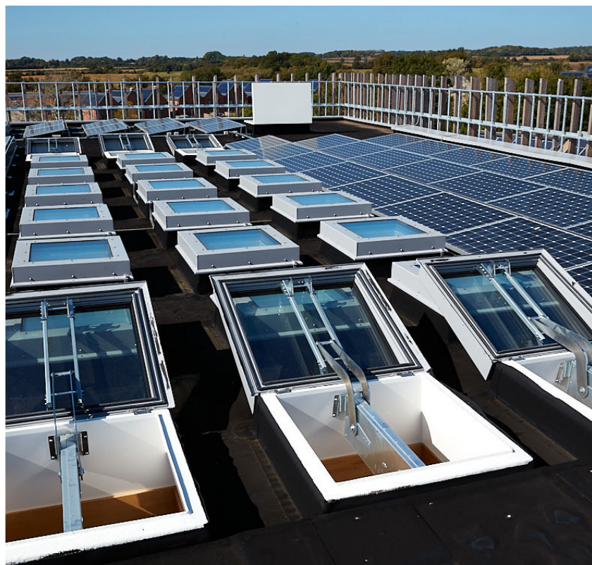
Smoke Lift Glass Skylight FE
