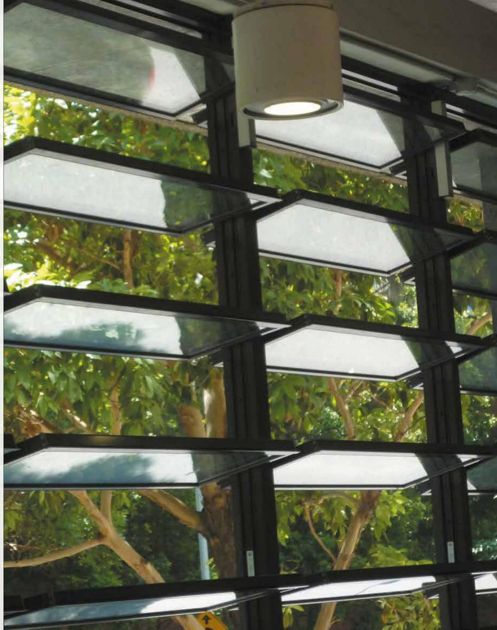
Picture: NTL ISO 24 BT50 louvre window fitted into a façade of an assembly hall.
