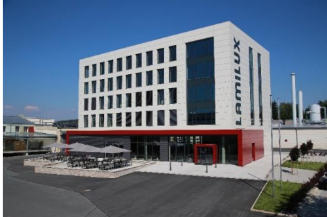
The LAMILUX administration building in Rehau, Upper Franconia - the headquarters of the family-owned company
