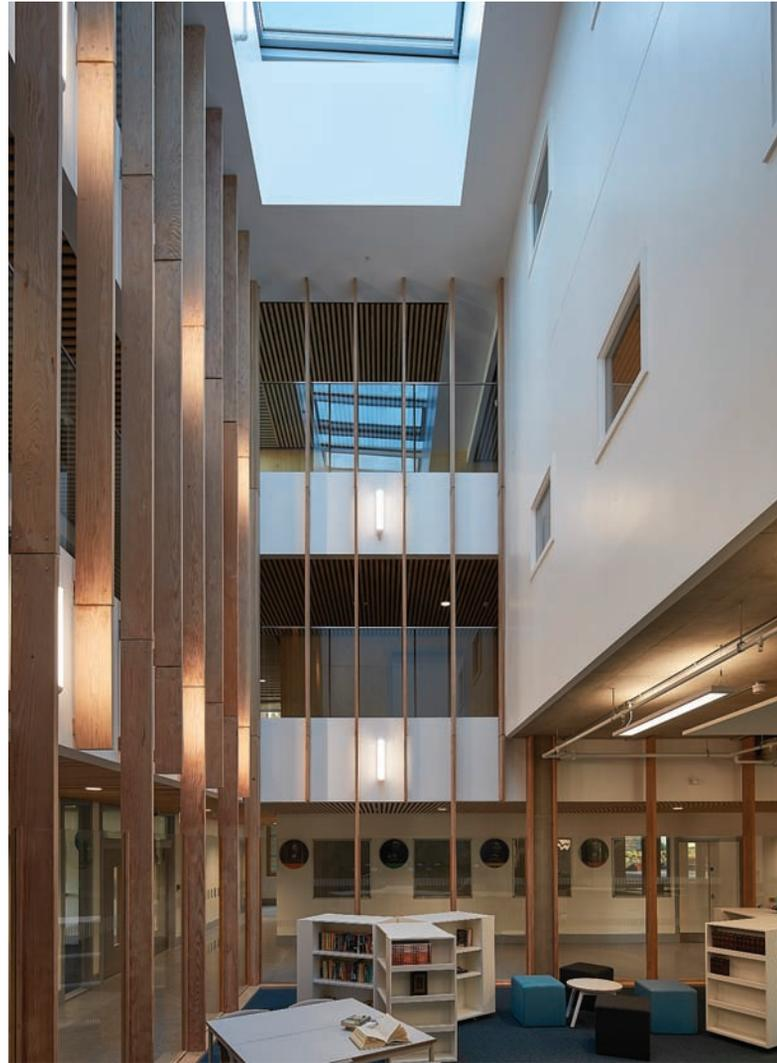
LAMILUX worked with main contractor Willmott Dixon to achieve the required light and solar performance. The triple glazed rooflights were specified with a toughened neutral high performance coated outer pane to provide comfort within the building, whilst achieving impact safety to CWCT TN92 Class 2 U-values and air-tightness values, according to the Passivhaus certificate – verified during the detailed design phase of the project.
