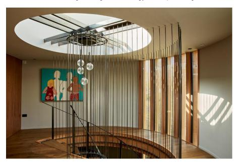
Three of the five skylights span an impressive 2500mm diameter to give plentiful natural daylight with a daylight size diameter of 2200mm. To achieve this non standard size, a special upstand was designed to support the rooflights.
