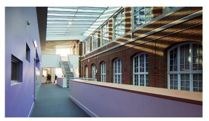
High performance glazing was essential to reduce solar heat gain and heat losses. Pilkington Suncool 70/35 was specified. 40 No fixed glass panels, each measuring 1.2 x 2.9m and weighing 150kg were used to reduce the buildings energy consumption, without compromising the daylight intake.
