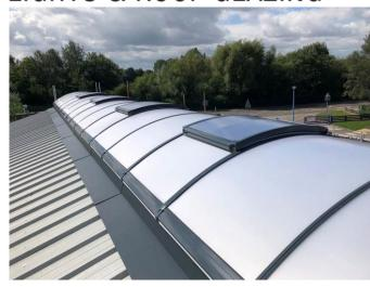
The LAMILUX U.K Ltd installation team recently completed a school refurb project in York, where they installed an incredible 65 meter long X 2.4 meter wide LAMILUX Continuous Barrel Vault Rooflight.
