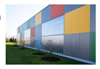
New construction of a production hall for electric motors with LAMILUX systems in the façade and on the roof for optimum daylight
