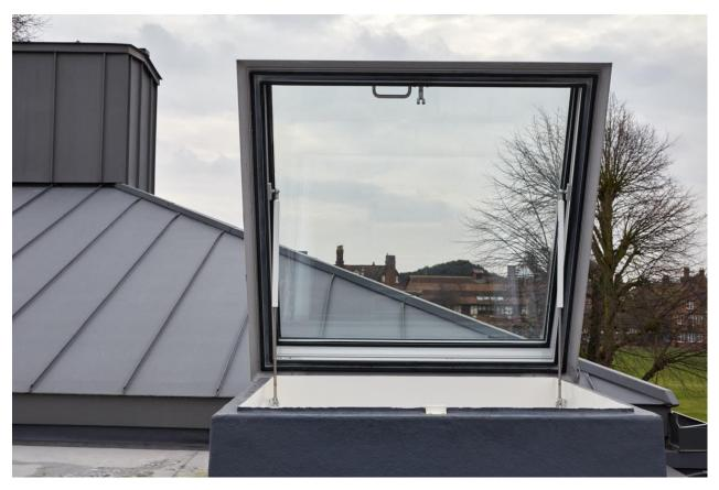
It was imperative that all rooflights met specific acoustic and thermal performance requirements, specific to their location on the roof. The rooflights supplied, featured effective glazing sound insulation values of up to 45dB. This performance, which is certified to EN ISO 140-3, was tested and approved by an acoustic consultant.
