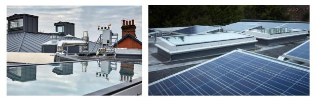
As standard, LAMILUX access hatches are pre-assembled to the GRP upstand, therefore a special lipped kerb was designed, to enable the contractor to complete the roof and seal the upstands before our upstands were installed. Grey frames (RAL 7047 – Telegrey 4) were chosen to tie in with the theme of the grey roof membrane.
