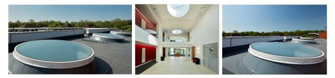
Each skylight measures a roof opening size of 2500mm diameter, offering a striking light size of 2200mm and an impressive 80% light transmission value, thus adding a generous amount of natural daylight to enrich the interior.
