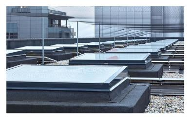
The local environment contained high chloride levels, due to the nearby sea, which meant that careful consideration to possible corrosion of the rooflight framework had to be considered. To eliminate this possibility, the aluminium frames were coated in a special anti-filiform treatment which was additionally powder coated to Anthracite Grey – RAL 7016.
